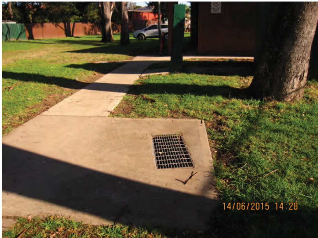
Rear park - Council's pit in the park
